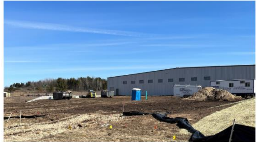
Parco Windows - completed
