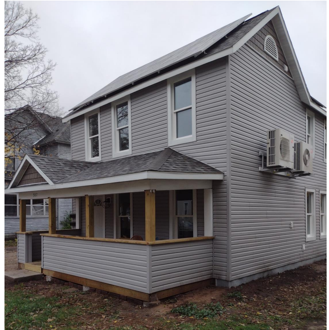
Duplex with Solar & Heat Pumps
